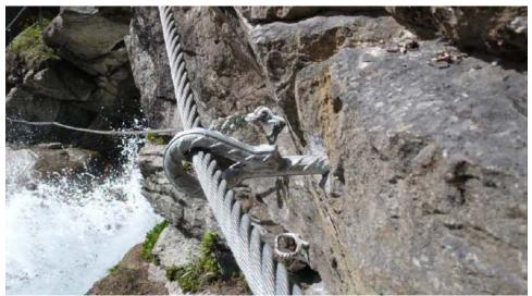
**Fig 16** Rebar eyebolt in a classic east-alps tensioned installation. The inner surface of the eyebolt is smooth and free of burrs.
