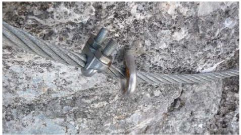
Fig 17 Cable clamps on either side of an intermediate anchor limit wear.
