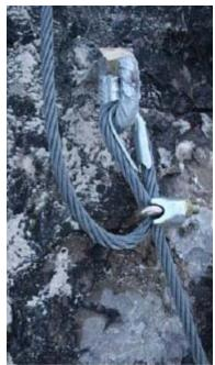
The French system with cable loops in eyebolts
